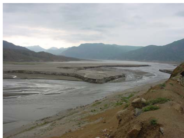
Figure 5. Sediment accumulation at the upstream end of Reservoir Gallito Ciego.
