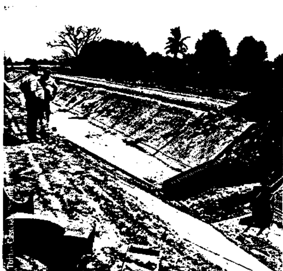
An irrigation channel being lined with concrete, Sinaloa Revestimiento de canal de riego con concreto, Sinaloa
