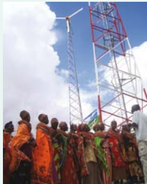
Wind turbine powering a Safaricom base station.
